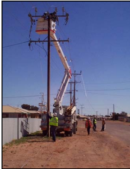
Distribution team at work on overhead lines
